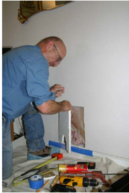
Remove interior piece of drywall & save to temporarily fill the hole.
