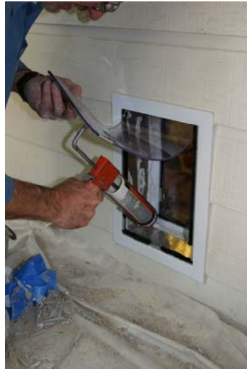
Apply the construction adhesive directly to the sides and bottom of tunnel.
