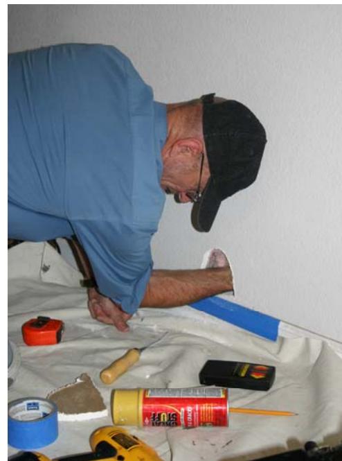
Look and feel for obstructions through a small hole before you cut out the entire hole for the pet door
