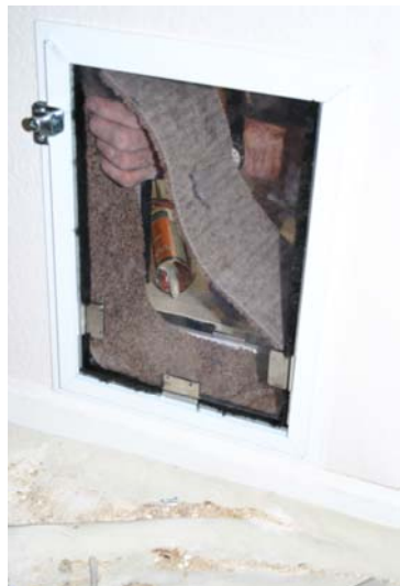
After cutting, dry fit the carpet first to verify measurements.
