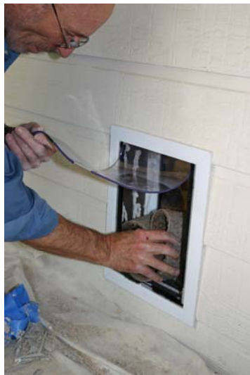
Roll the two ends of the carpet inward and place in bottom of tunnel.
