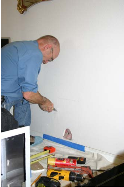
Cut the opening with a drywall saw.
