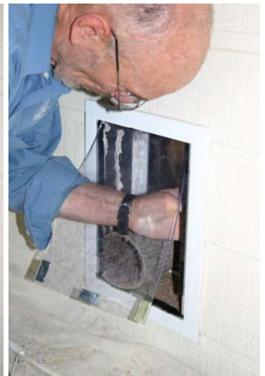
Carefully unroll the carpet pressing firmly against sides & bottom of tunnel.
