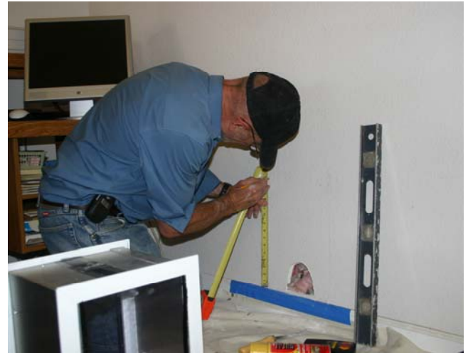
Measure and mark the hole carefully, making sure it is square and level.
