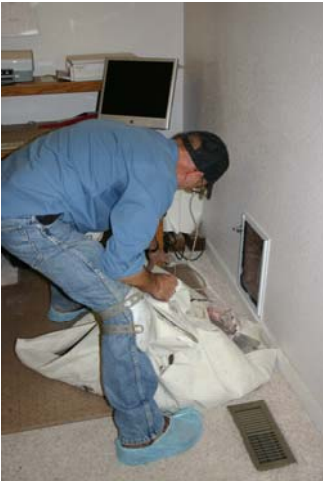
Wrap up any installation debris in the drop cloths for easy removal.
