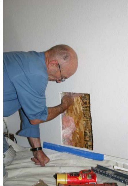
Push the insulation into the wall out of the way
